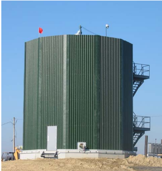
Left: Sessil trickling filter at JBB with custom colored paneling to match the existing facility. Above: Motorized galvanized rotary distributor for even distribution of the wastewater onto the Sessil media.
