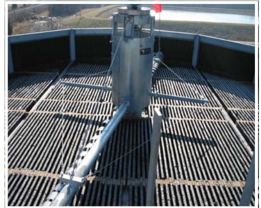
Left: Sessil trickling filter at JBB with custom colored paneling to match the existing facility. Above: Motorized galvanized rotary distributor for even distribution of the wastewater onto the Sessil media.
