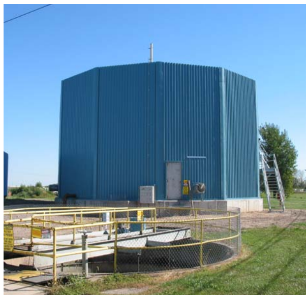
Left: Sessil trickling filter at USG with custom colored paneling to match the existing facility. Above: Motorized galvanized rotary distributor for even distribution of the wastewater onto the Sessil media.
