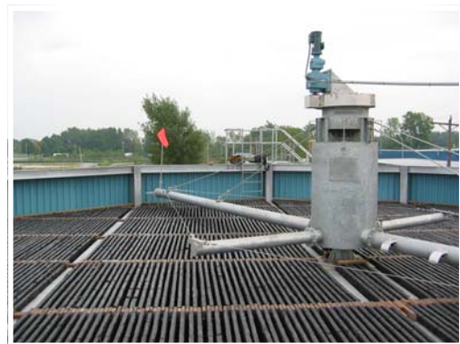
Left: Sessil trickling filter at USG with custom colored paneling to match the existing facility. Above: Motorized galvanized rotary distributor for even distribution of the wastewater onto the Sessil media.
